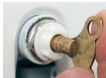
Figure: Bleed valve and key
