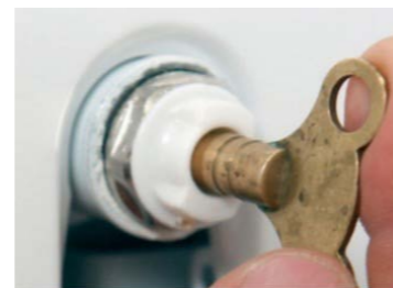
Figure: Bleed valve and key
