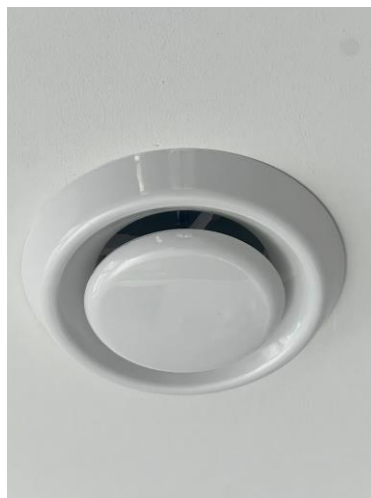
Kitchen and Bathroom Vent
